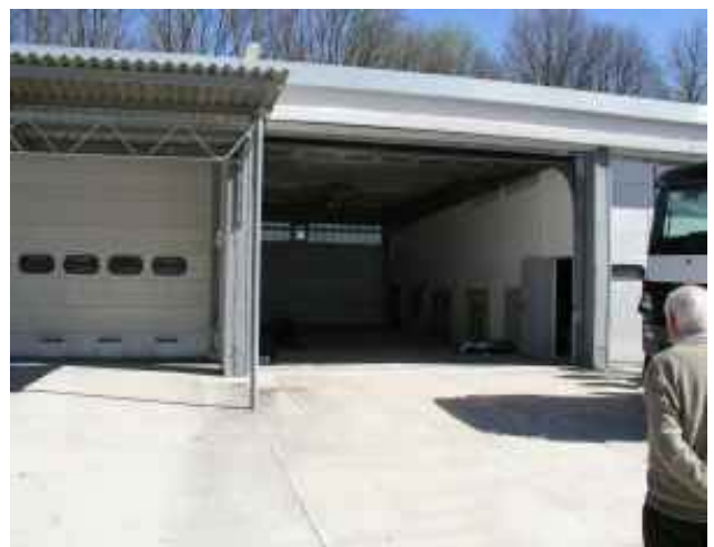
fig. 5.3 - 1 Hall 17 before its transformation into test room
